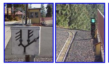
The new signal system installed at Central Station can be run by selector box as shown on the left or from a dispatcher working the tower seen in the distance. Steve Panzik lent the group a couple of his full size signals and they are really impressive. Check out the Tower Statistics listed below. This is one of the side benefits to the computer oriented signal system, pretty cool!
